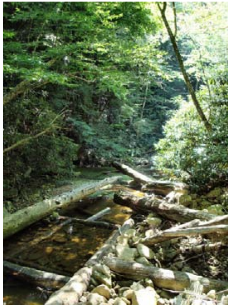
Splash dam remains on the main stem of the Middle Fork Williams River. This is the river right side of the dam looking up a portion of the Middle Fork.
