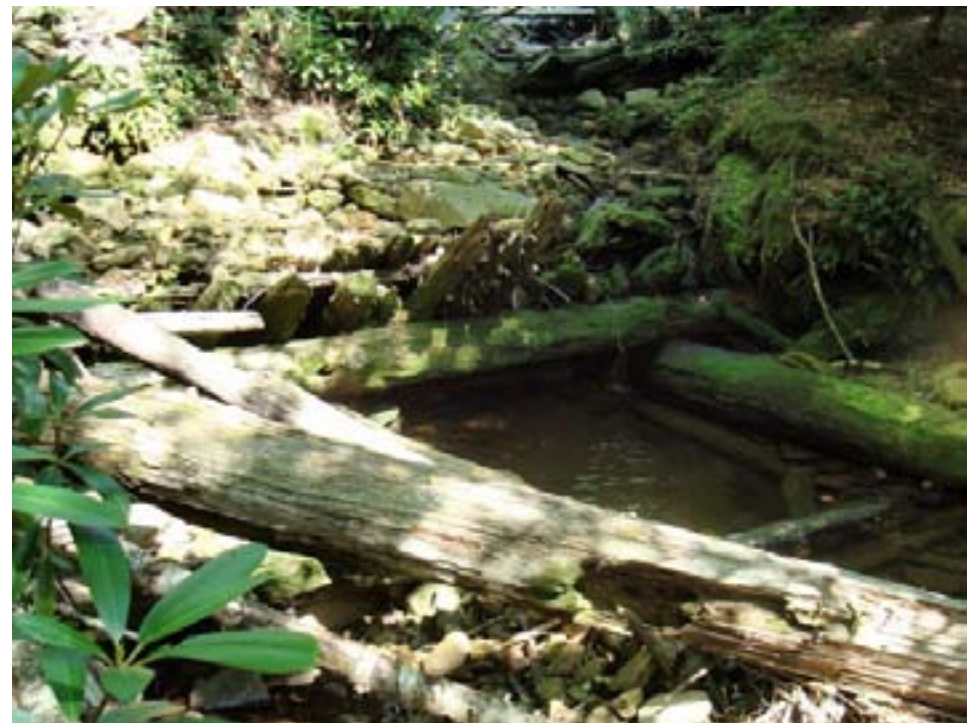
Splash Dam remains where McClintock Run enters the main stem of the Middle Fork Williams River. See the log structure and the upright boards on the upstream side.
